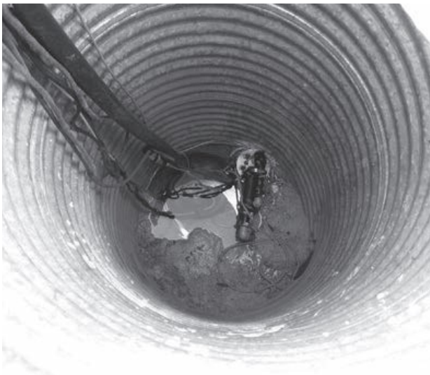
Drilled well in a pit.
