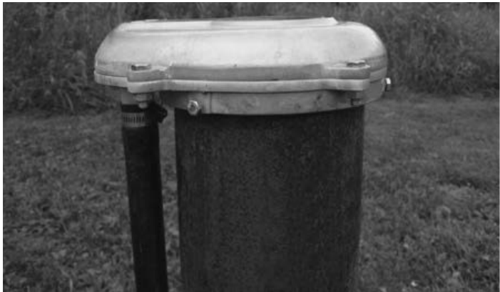
Above: Vermin-proof cap for dug or bored wells. Credit: Manitoba Water Well Association Below: Vermin-proof cap for drilled wells.
