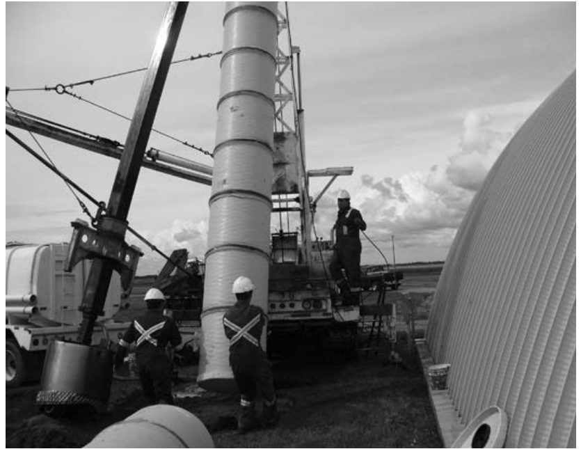
Bored well construction
